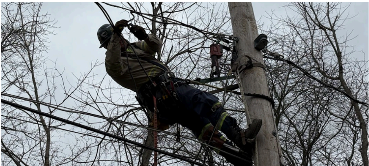
Electric crew repairing damage from the recent wind storm.
